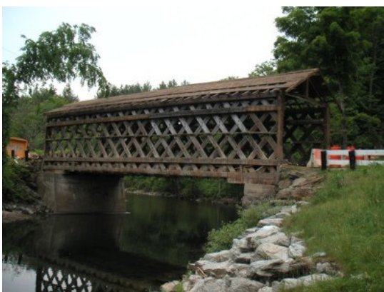
Comstock Bridge, near Montgomery, Vermont.
