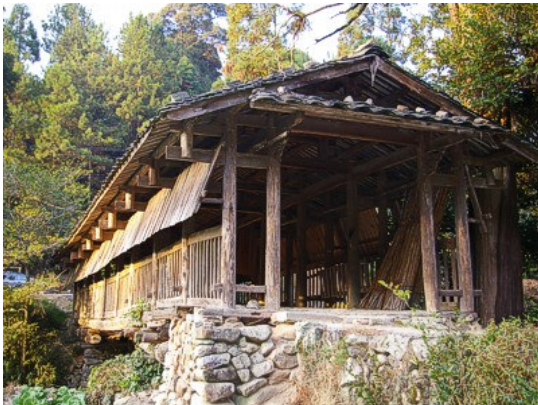
Baogong bridge near Pingnan, Fujian province.
